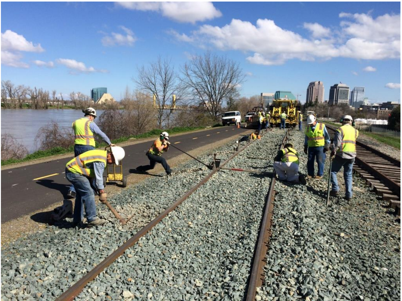
The MOW Team track-raise crew is a well-oiled machine!
