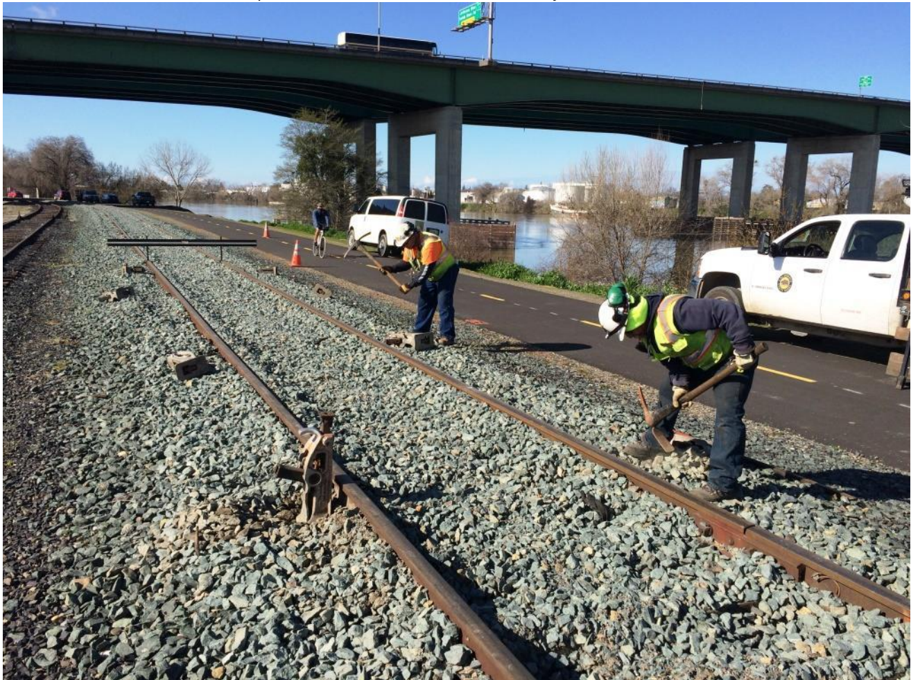
Mike F. and Joe dig pockets into which jacks will be set
