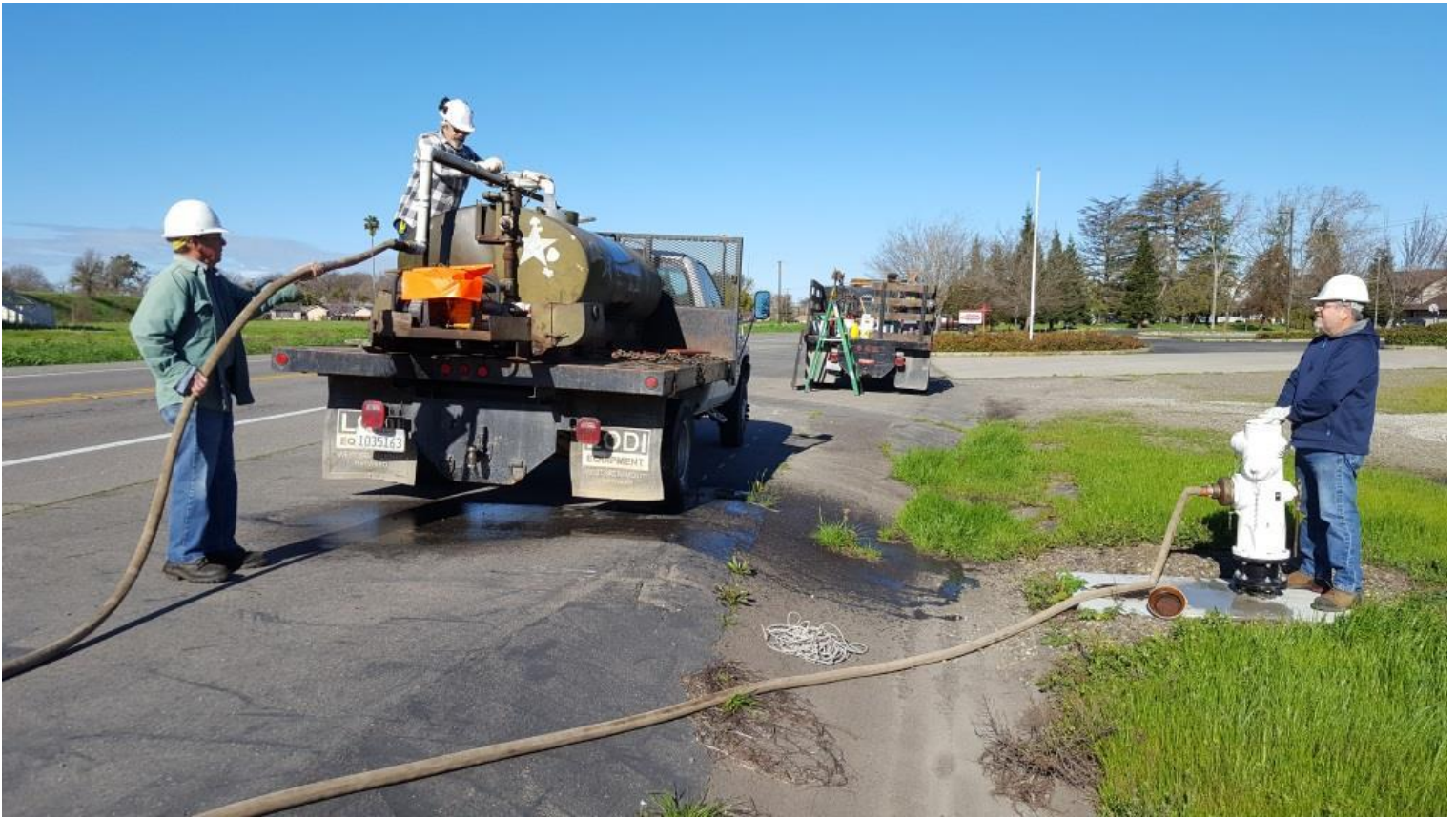
Mike T., Ed, and Steve W. fill the 400-gallon water tank (with permission, of course)
