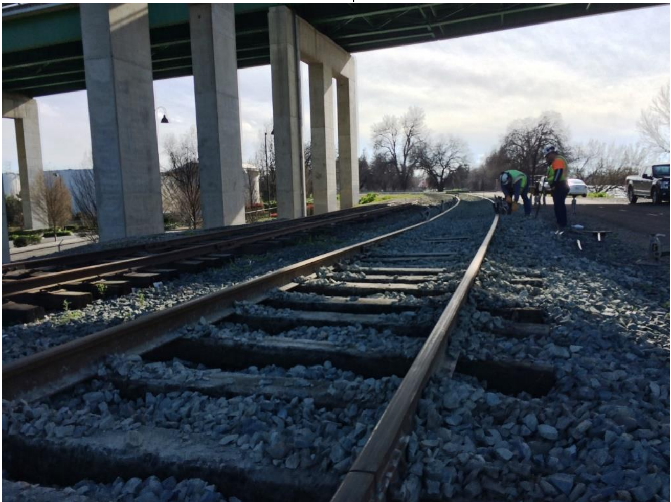
Frank and Mike H. build the run-off at the end of the raise
