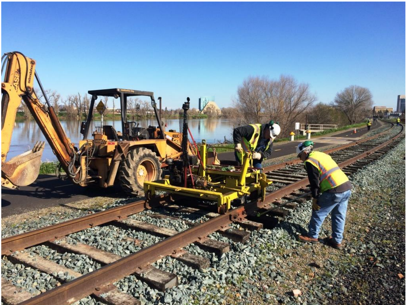
Chris operates the rail-lifter as Mike W. places tie-plates
