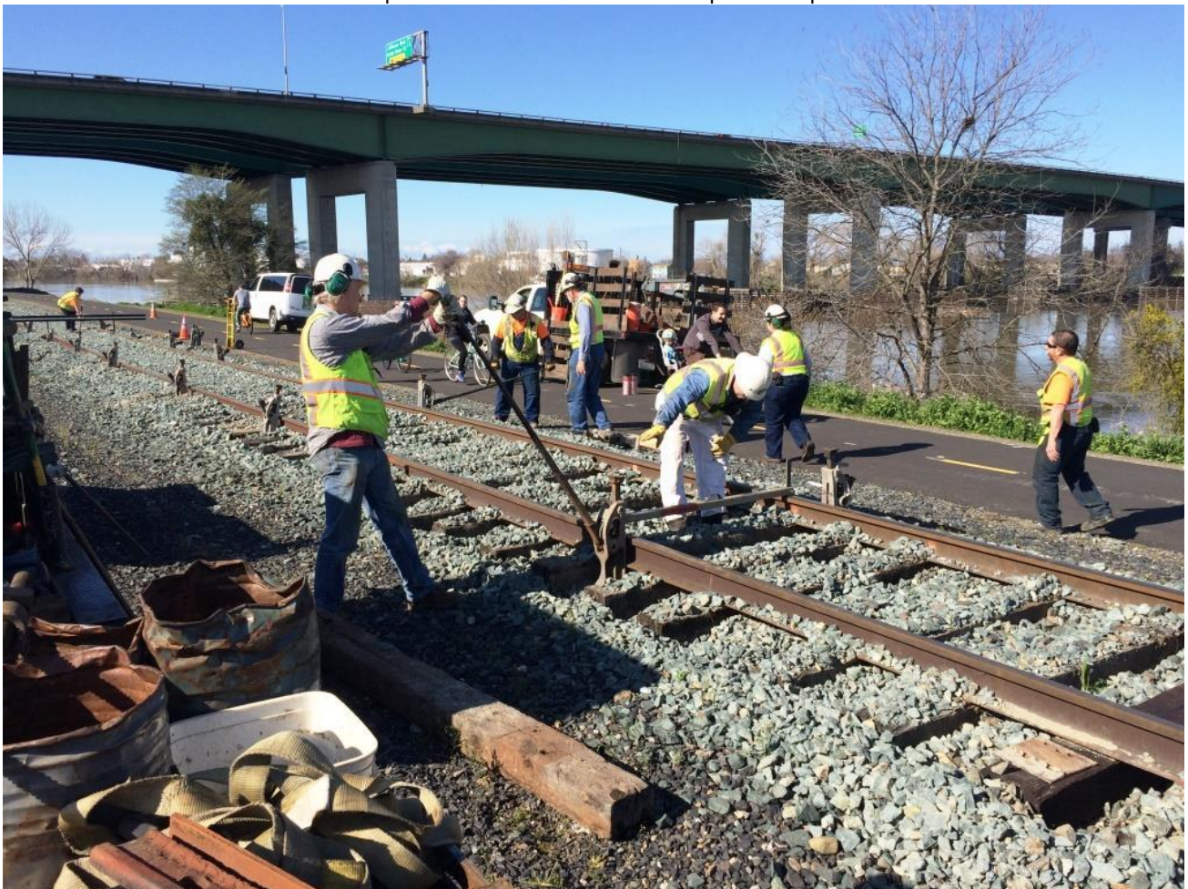
Mike H. checks the track-level and guides Steve N. as he raises the jack
