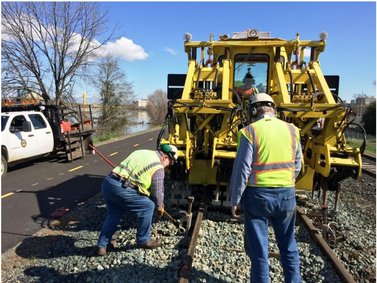
Frank removes a jack as Mike F. in the tamper, guided by Alan, tamps the track to the new level
