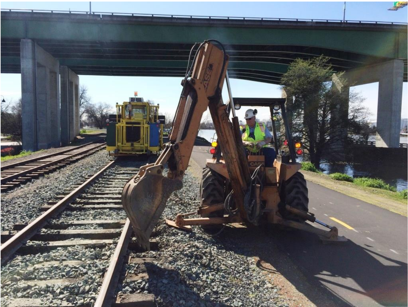
Chris on the back-hoe pulls another tie
